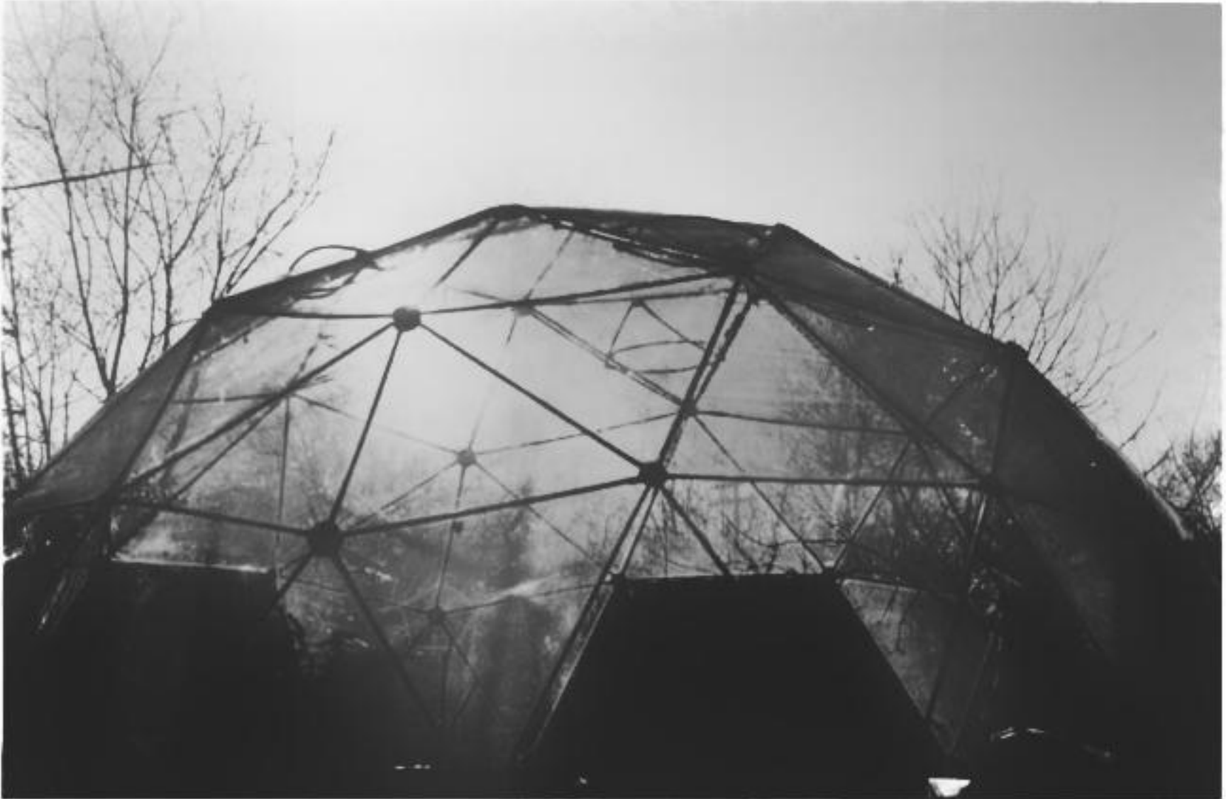
FIGURE 39-5 Prototype bioshelter. A geodesic dome housing fish and vegetable modules. Photo by J. Todd.
